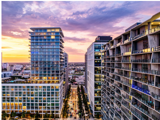
Water Street, Tampa, FL
